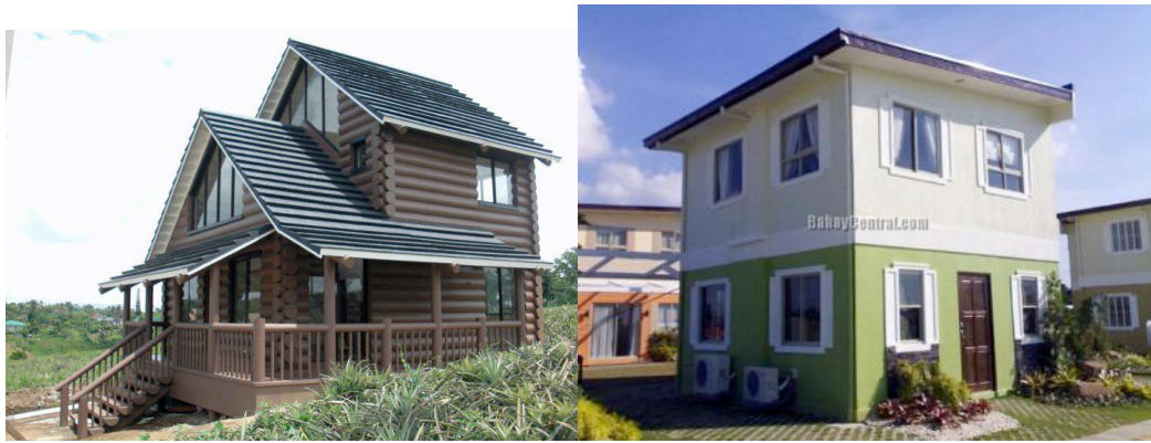
Figure 3. A “log cabin” that’s actually made of concrete built on an open field (left) and a block design requiring multiple air-conditioning units (right).
